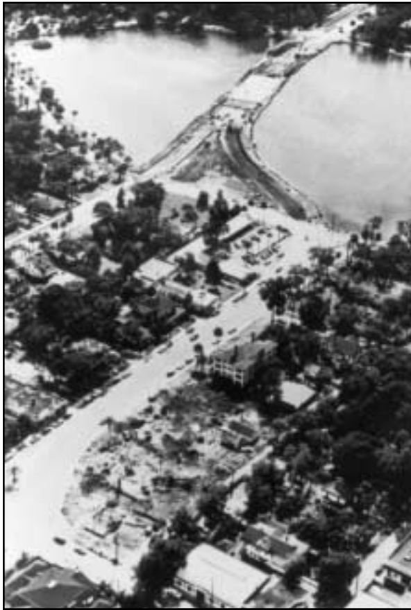
Looking south across Lake Lucerne in 1955 during construction of the Orange Avenue causeway.
